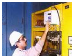
Fig 2. Local equipment in electric house;
